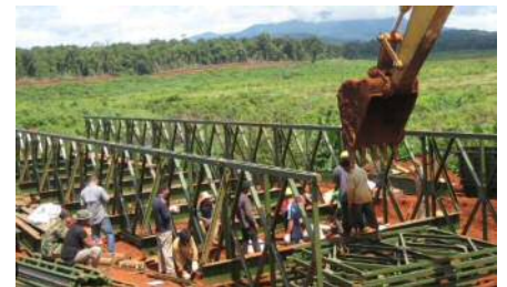
Fabrication at the site
