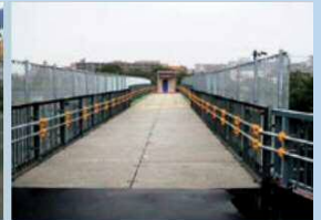
Temporary bridge for pedestrian walkway
