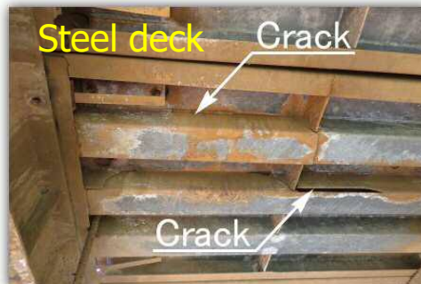
Fracture and Fatigue cracks due to heavy traffic
