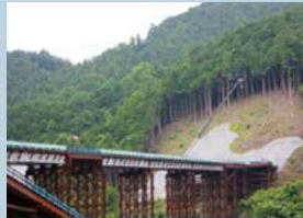
Temporary bridge for construction road
