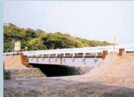
Emergency bridges in times of disaster
