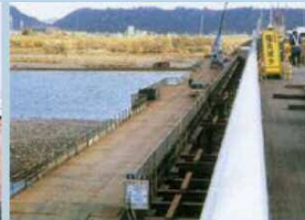
Temporary Jetties for cranes and other work
