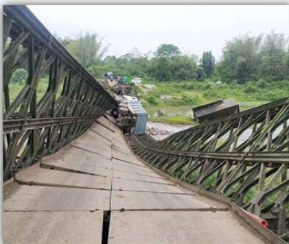
Bridge collapse due to buckling of steel members
