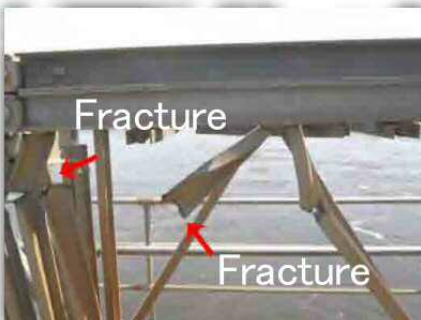
Fracture and Fatigue cracks due to heavy traffic
