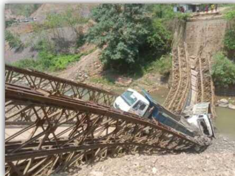
Bridge collapse due to buckling of steel members
