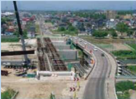
Reroute for replacement construction
